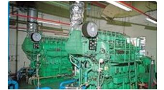
Diesel engines for emergency pumps
