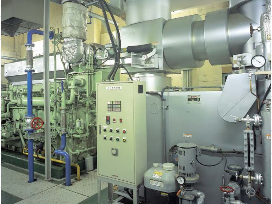
Exhaust gas boiler
